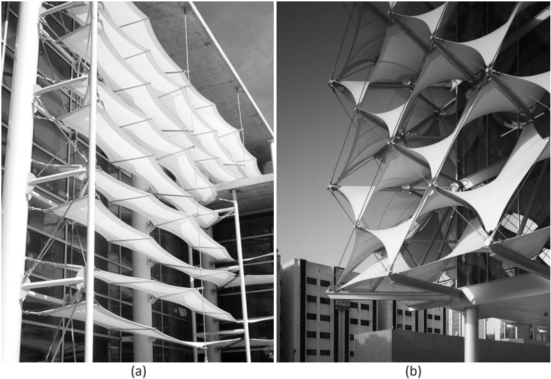
Figure 4. Fabric façade for sun and wind protection. (a) Fabric façade of the Mesa Arts & Entertainment Centre, Arizona, USA. (Source: https://www.fabritecstructures.com ) (b) Fabric façade of National Library in Riyadh, Saudi Arabia. (Source: https://s-media-cache-ak0.pinimg.com )
