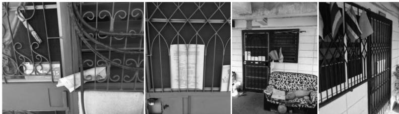
Figure 3. Steel grilles installed in front of windows and doors, increasing security of residents.
