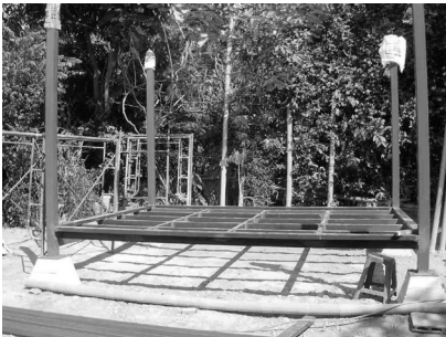
2. Install column and beam.
