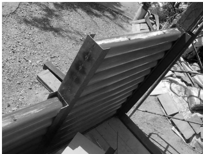
4. Insert the artificial log on stud.
