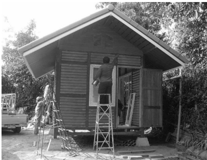
6. Install roof structure and door.
