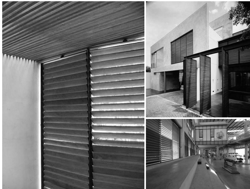
Figure 4. Exemplary projects applying the jalousies hardware set as low-cost outdoor shading device, designed by co-author, Srisak Phattanawasin; 4C House (2007) on the left and the top right, and Automotive Engineering Workshop Building at Thammasat University (2015) on the bottom right.
