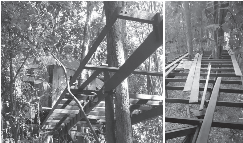
Figure 11. Floor frame and flooring installation.
