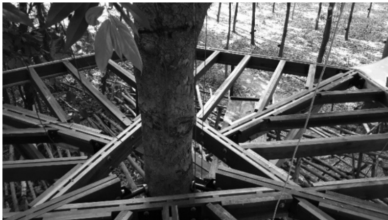
Figure 6. Floor framing.
