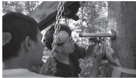
Figure 10. TAB and Tri-beam installation.
