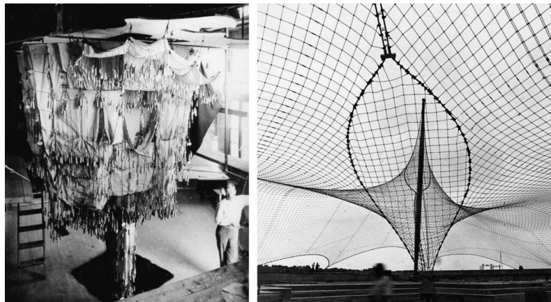
Figure 6. Funicular and self-stressing form systems: (a) hanging model for the Church of Colònia Güell made by Gaudi (Martin, 2015); (b) German Pavilion at Montreal in 1967 designed by Frei Otto (Detail 6, 2000).
