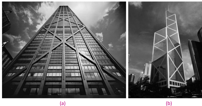
Figure 13. Traditional diagonal bracing of high-rise buildings: (a) John Hancock Center in Chicago (Stoller, 2021); (b) Bank of China Tower in Hong Kong (Fu, 2019).
