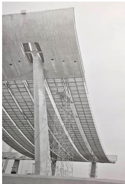
Figure 4 The concrete sheet of Washington Dulles International Airport under construction, Eero Saarinen. 1961. (Bell & Buckley, 2010, p.59)
