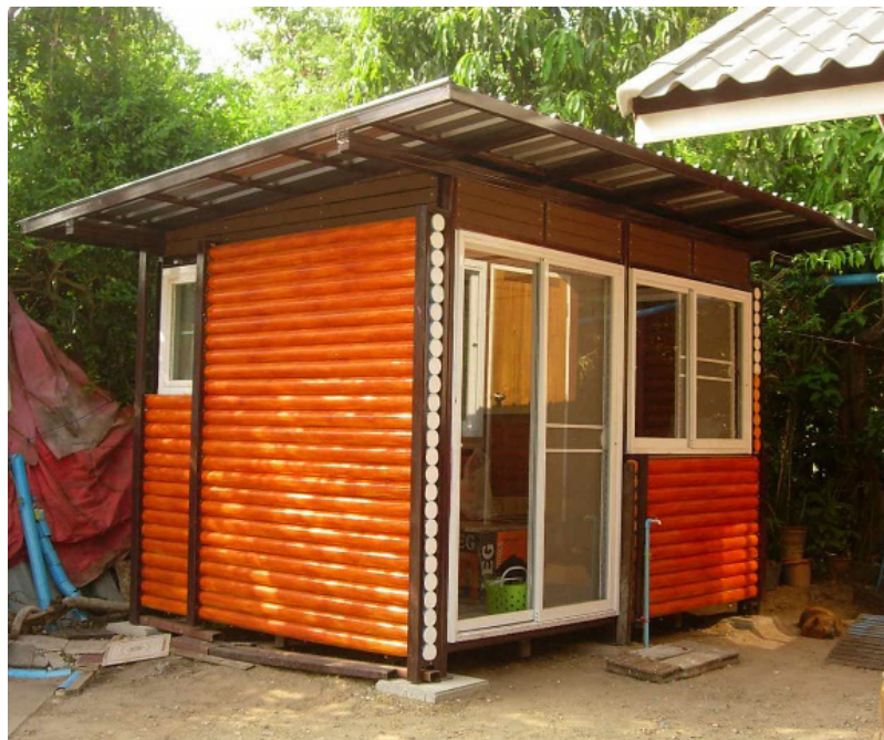
Figure 1 Sangrutsamee and Khamput's (2018) shelter from prefabricated PVC pipe panels
