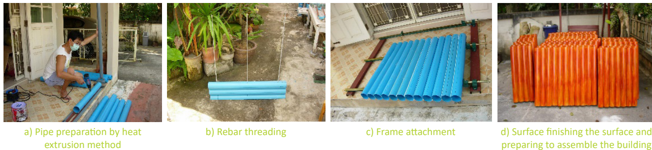
Figure 3 Assembly of prefabricated wall panels from PVC pipes
