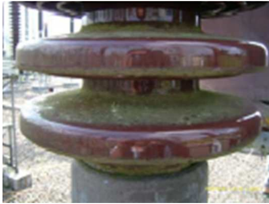
Fig.28: The sticky pollutant on the insulator surface of Kamojang switchyard
