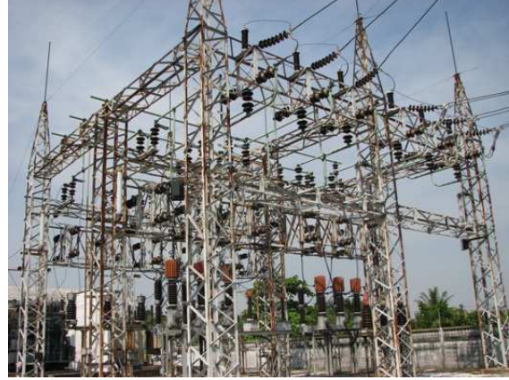
Fig.1: Bangkrachao Primary Outdoor Type 69/12-24kV Substation
