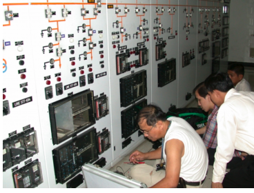
Fig.4: Installation of electricity recorder of overhead transmission lines [22].
