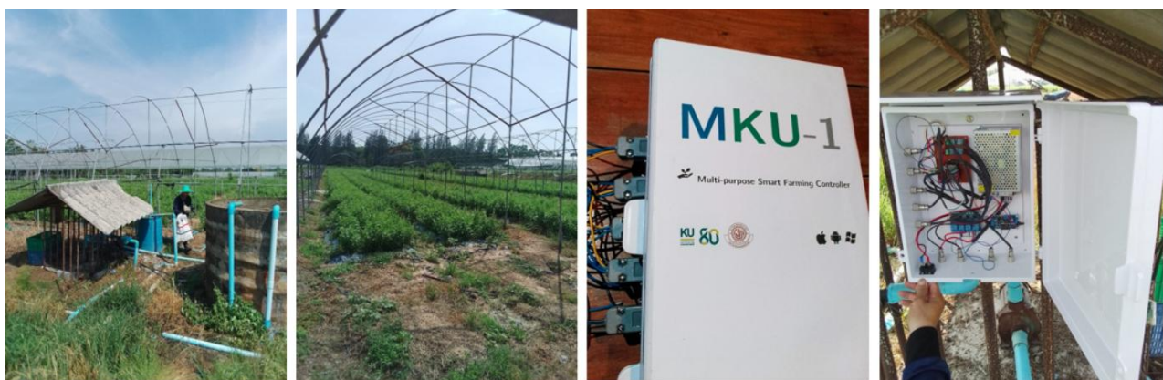
Figure 3. The experimental site for system installation and the prototype developed and implemented in this paper
