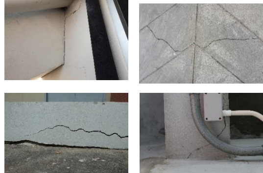
Fig. 1. Example images of cracks used in this study
