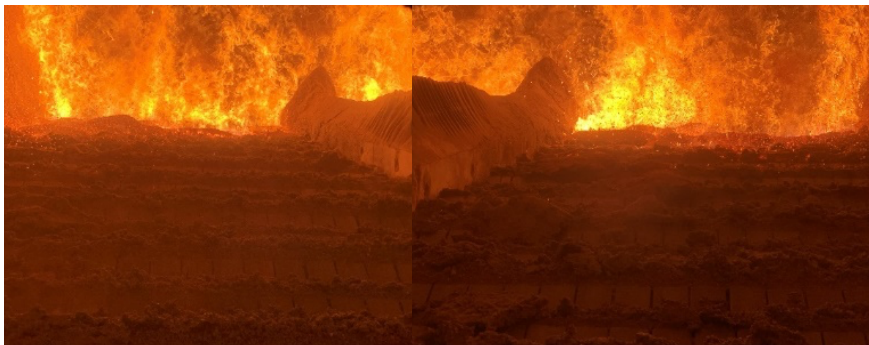
Fig. 14. The high combustion grate zone.
