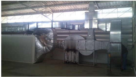
Fig. 3 fruit dehydration machine by biomass energy
