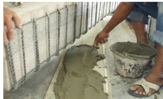
(c) Plastering mortar at the bottom face
