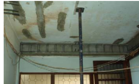
(a) Side-cover for edge beams
