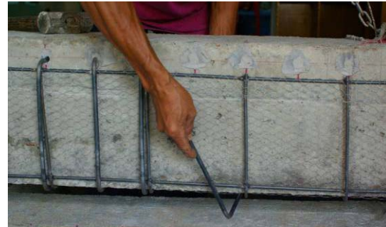
(b) Installing U-shape bars and skeleton steel
