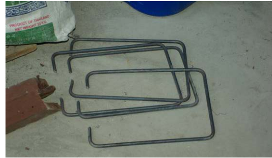
(a) U-shape external web reinforcements
