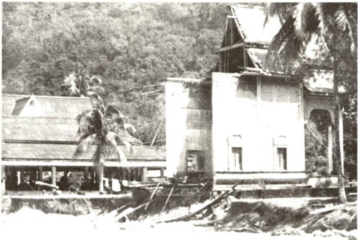
Fig. 2 Typical Landslides and Flooding at Ban Krathun (Above) and Severe Damages Due to Floods and Debris Flow at Ban Kiriwong (Below), Nakhon Sri Thammarat Province
