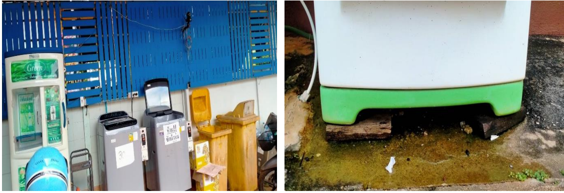
Figure 4. Typical location of drinking water vending machine
