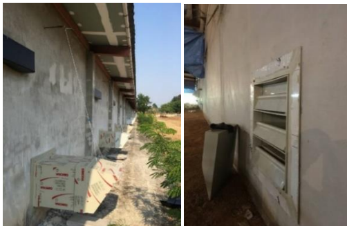
Figure 3 Installation of air inlet equipment and feature
