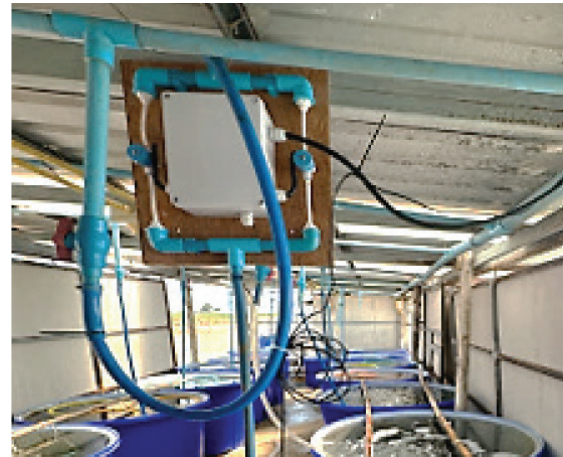
Fig. 4. The design of the valve controls the oxygen supply to the water for sea lettuce cultured process
