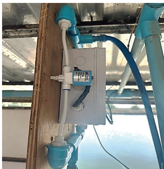
Fig. 3. The solenoid valve controls system
