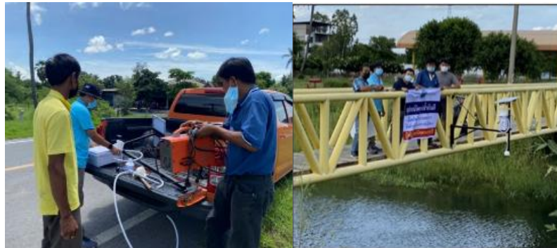
Figure 5 Installation of the automatic water level measurement tool.
