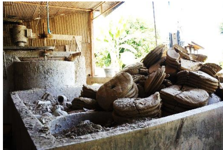
Figure 2. Condition of the tank and surrounding area of the slip-casting preparation area.
