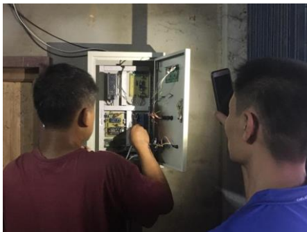
Fig. 13 Installing the first version of the IoT control box for mushroom plant
