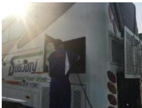
(b) Condensing unit cleaning up.
