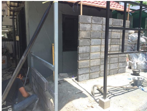
Figure 12. Testing the use of hollow concrete blocks by wall formation.
