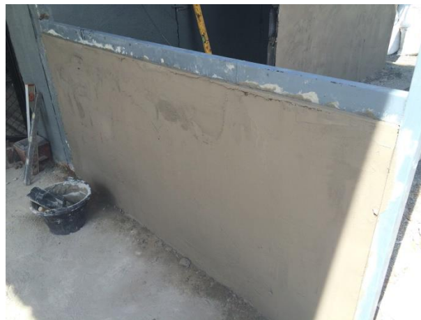
Figure 13. Hollow concrete blocks walls that have already been plastered.
