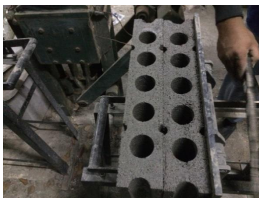
Figure 5. Hollow concrete blocks ready to be cured.
