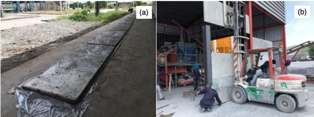
Figure 6. Production soundproof plate(a) and installation soundproof wall(b)
