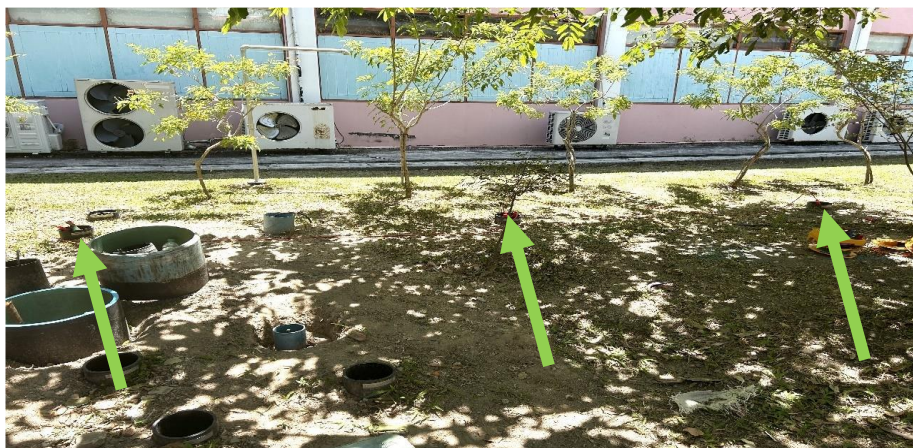
Figure 2. Three-core copper-clad steel straight earth resistance measurement
