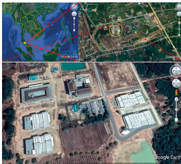
Figure 1. Satellite imagery of the study area shows the location of the proposed 1 MW solar PV rooftop installation.
