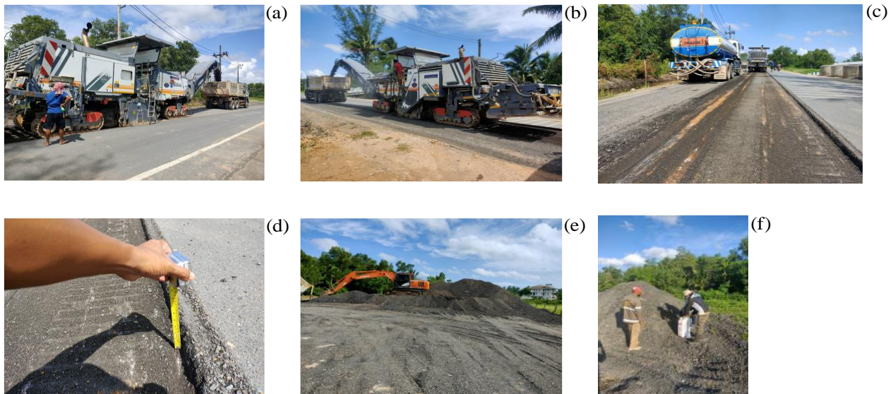
Figure 3. Collecting the RAP (a) milling machine (b) milling machine in operation (c) pavement after RAP peeled (d) depth of peeled surface (e) pile of milled RAP (f) collecting RAP
