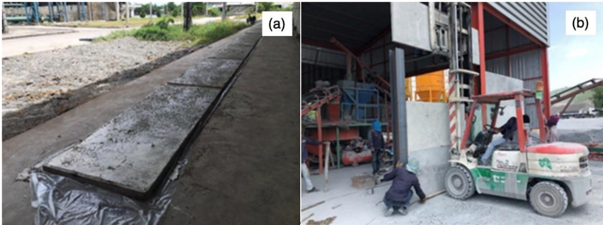
Figure 6. Production soundproof plate(a) and installation soundproof wall(b)
