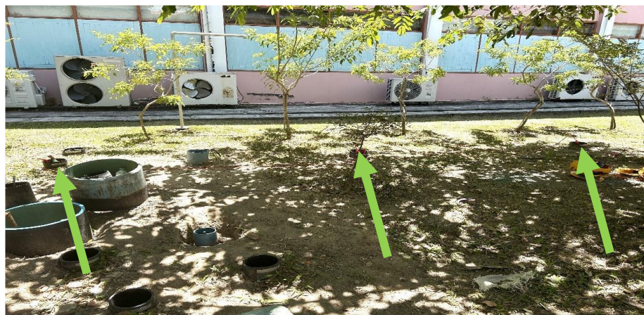
Figure 2. Three-core copper-clad steel straight earth resistance measurement
